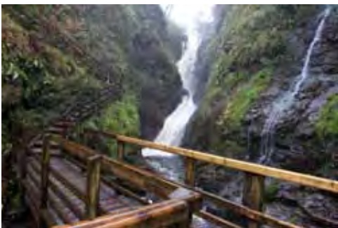
Repaired viewing platform at Waterfalls Walk
