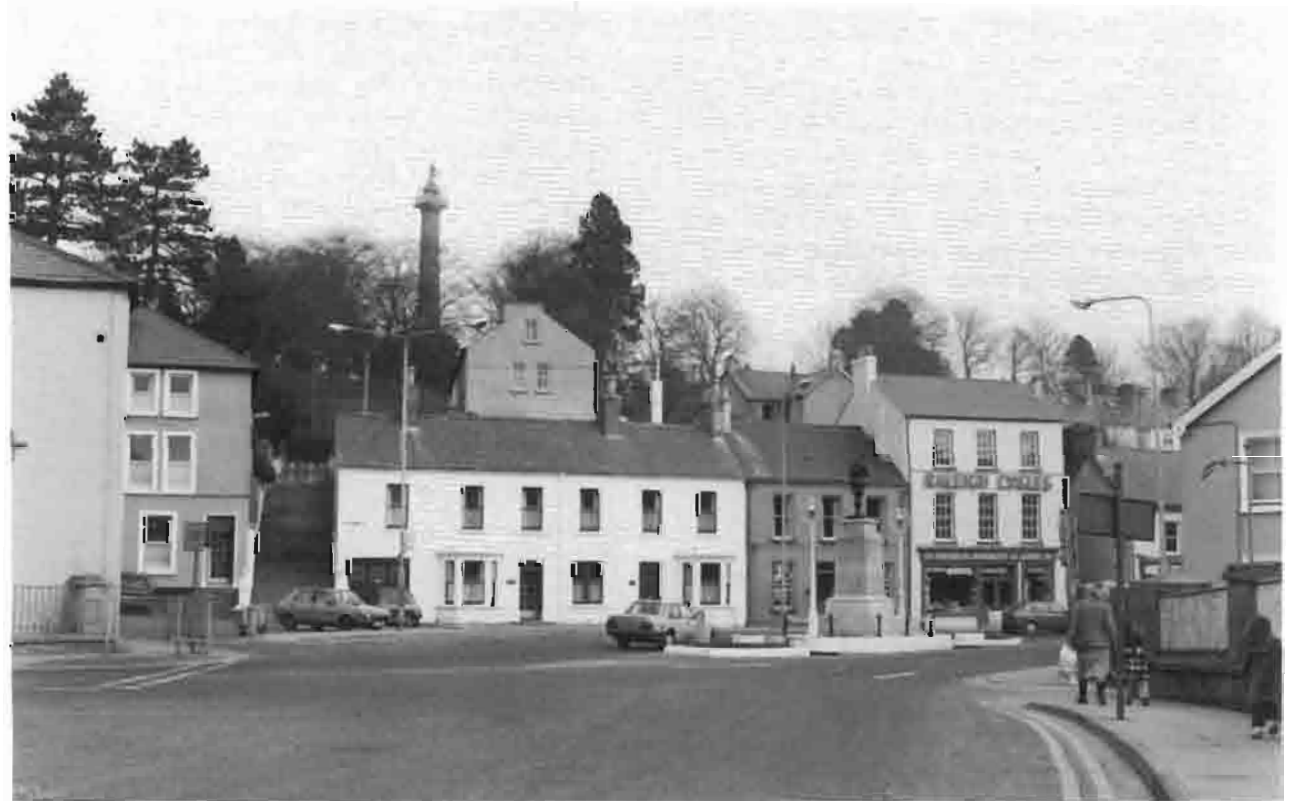
Belmore Street with its trees backdrop — the eastern end of the Conservation Area
