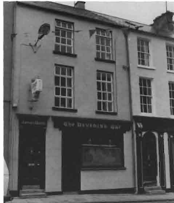
New shop and pub fronts adopting the traditional approach
