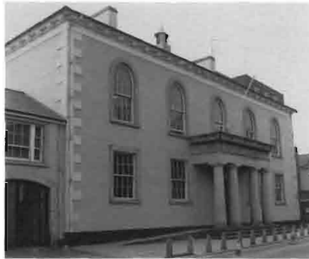
The Courthouse refurbishment scheme has created a considerable impact in the street scene
