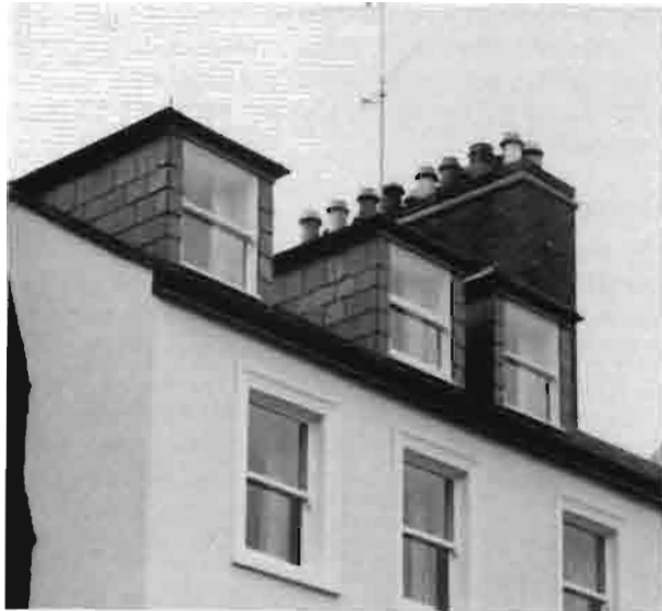
Dormer windows should be traditional in design and in scale with existing building
