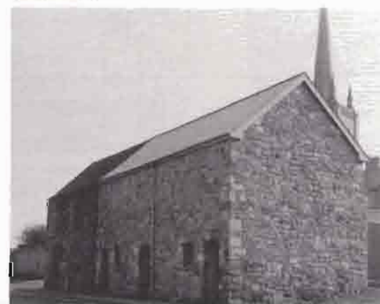
Refurbishment of backland building to provide public conveniences
