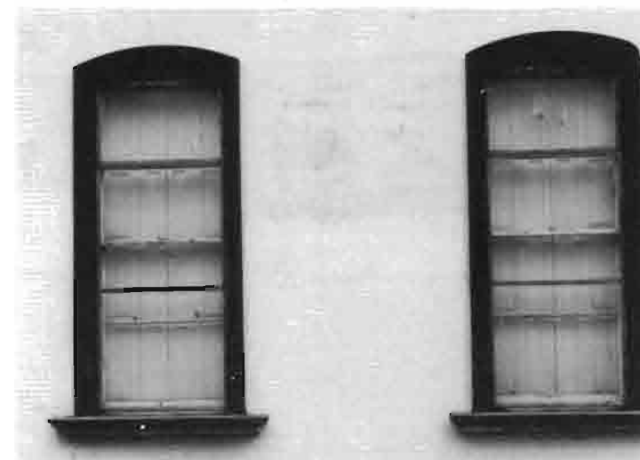
Two acceptable solutions to the problem of dealing with shutters. Shutters should form an integrated part of the shop front and should not project beyond the face of the building.
