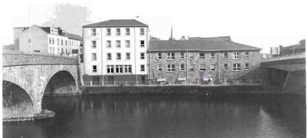
West Bridge House Anne Street — Traditional approach
