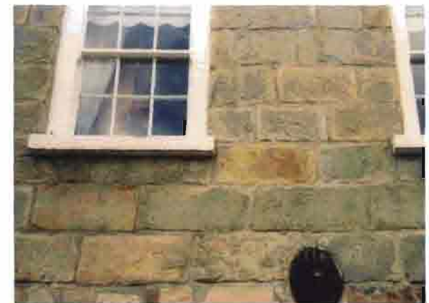
Squared sandstone, laid to courses
