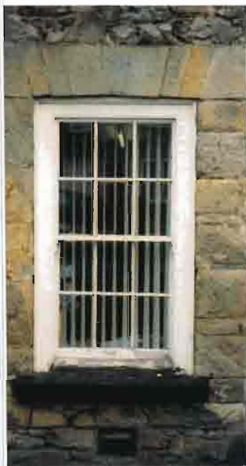
Original type window, with exposed sash boxes
