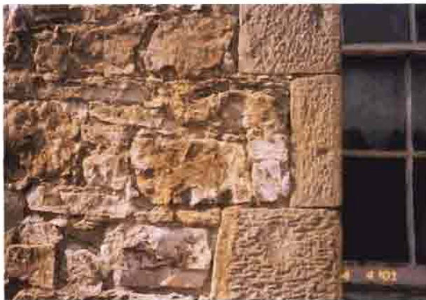
Cut stone, ashlar jointed window surround.
