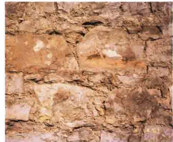
Rubble limestone walling
