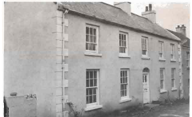
Contrasting colours or black or white are recommended for doors and windows and for features such as surrounds and quoins.
