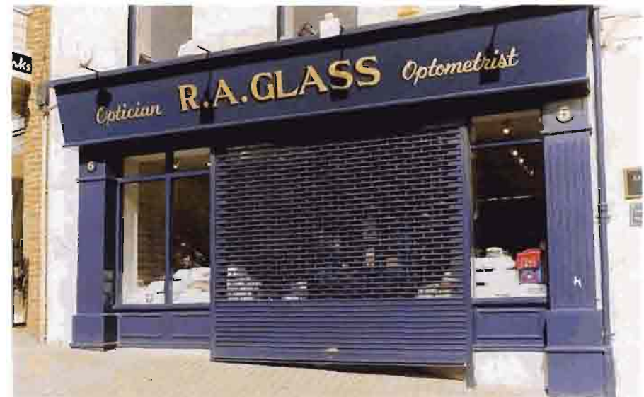
Acceptable Shutter detail ( 5 Market Place Carrickfergus)
