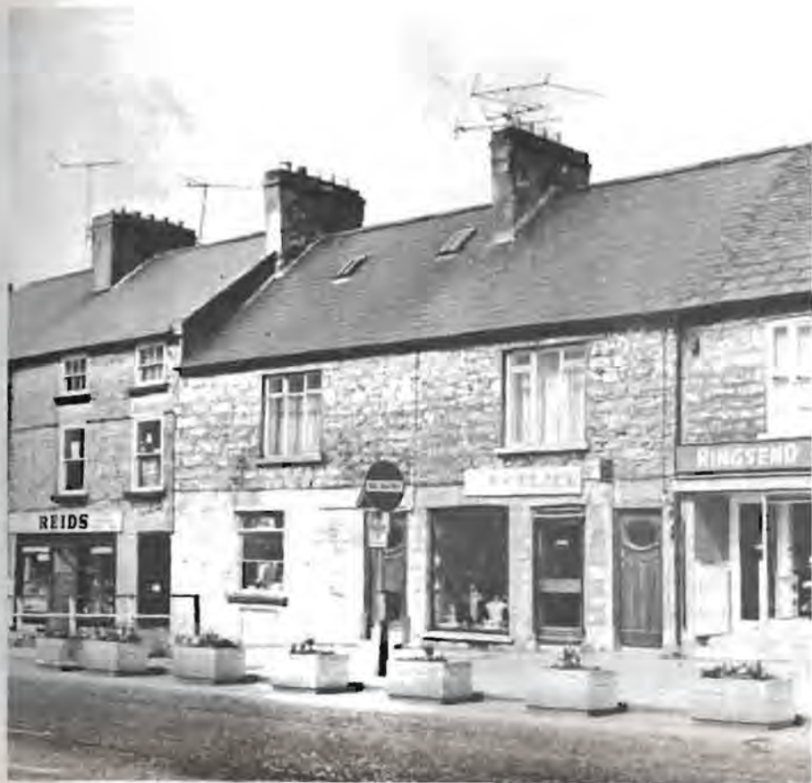
It is the repetition of regular, narrow frontage sites such as those in Barrack Street which contributes much to the character of the commercial core.
