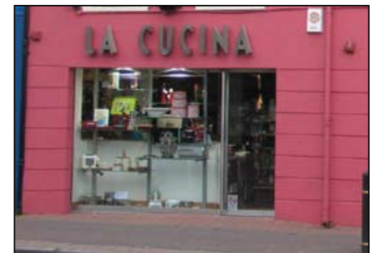
Shopfront, No. 63 High Street, Hollywood
