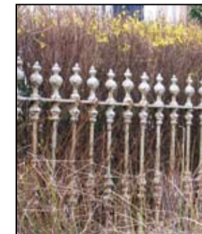
Cast iron railings
