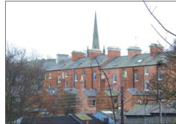
Roofs make a vital contribution to the character of the area
