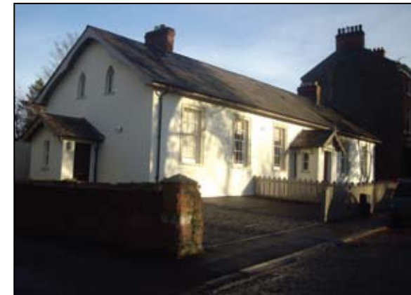
Hollywood Old School, Church Road, Hollywood (After refurbishment)
