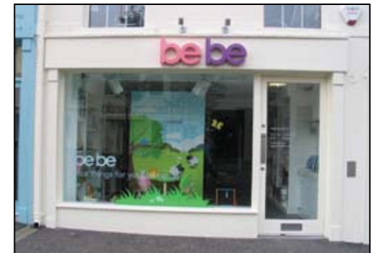
Shopfront, No. 6 Shore Road, Hollywood
