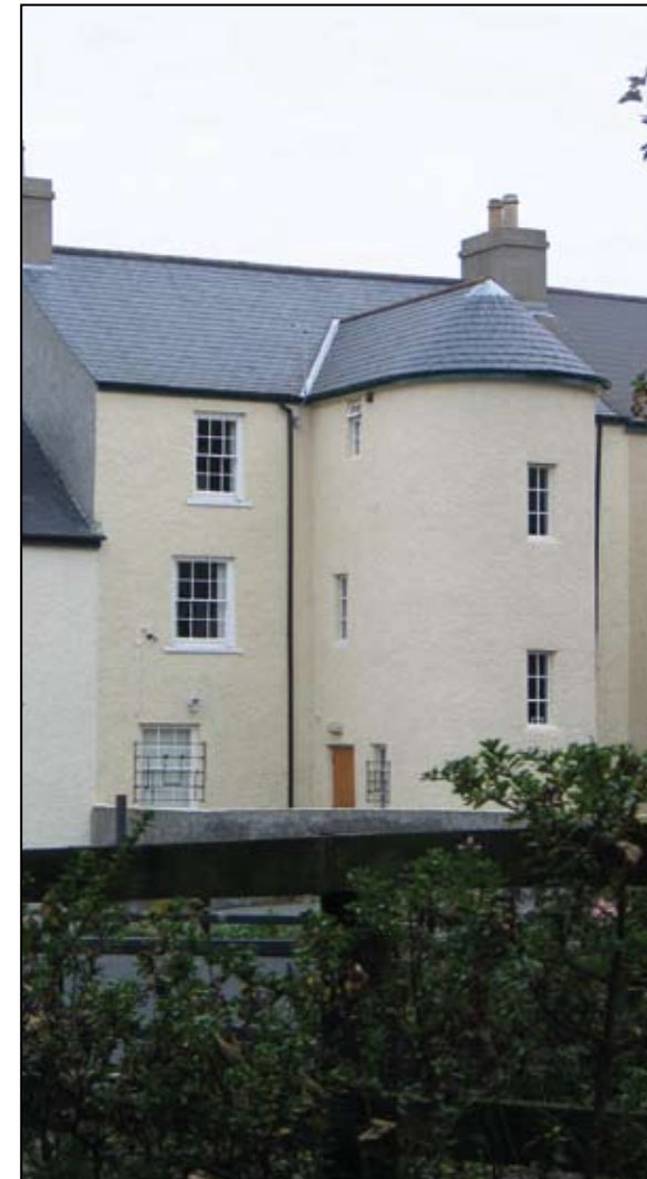
Rear staircase extension
