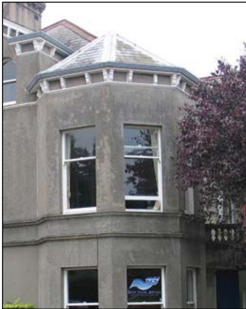
Octagonal turret, natural slate roof and lead roll-top hips
