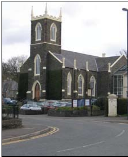
First Holywood Presbyterian Church
