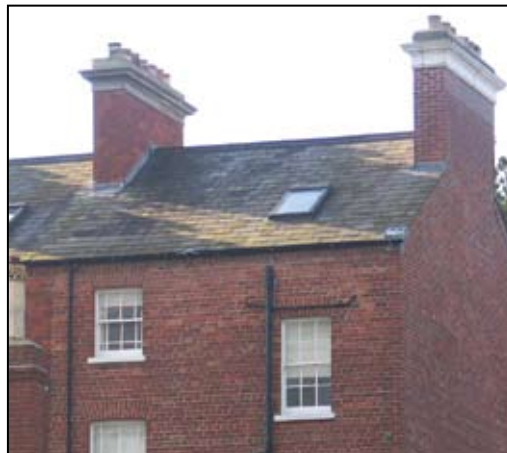
Gabled, natural slate roof with cast iron gutters
