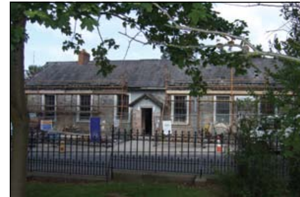
Hollywood Old School, Church Road, Hollywood (Prior to refurbishment)
