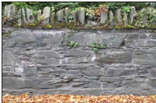
Stone walling, Victoria Road
