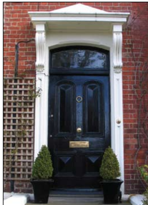
Four panel raised and fielded door with moulded surround
