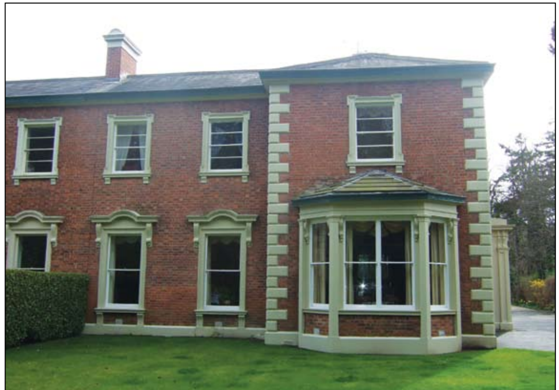
Hipped, natural slate roof
