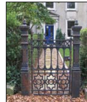
Cast iron gates
