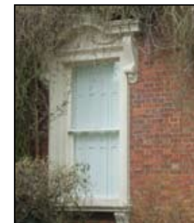
Moulded window surround
