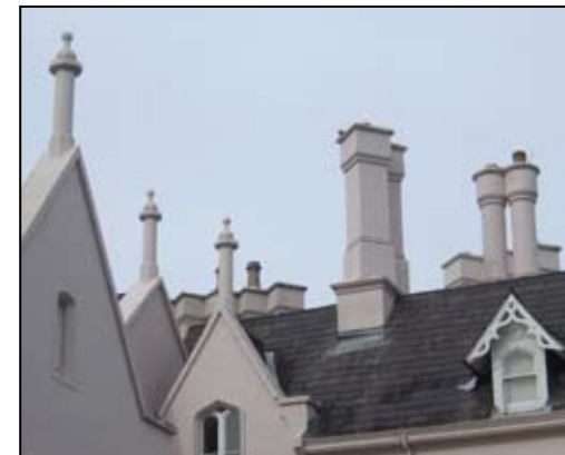
Finials and diagonally set coupled rendered chimneys
