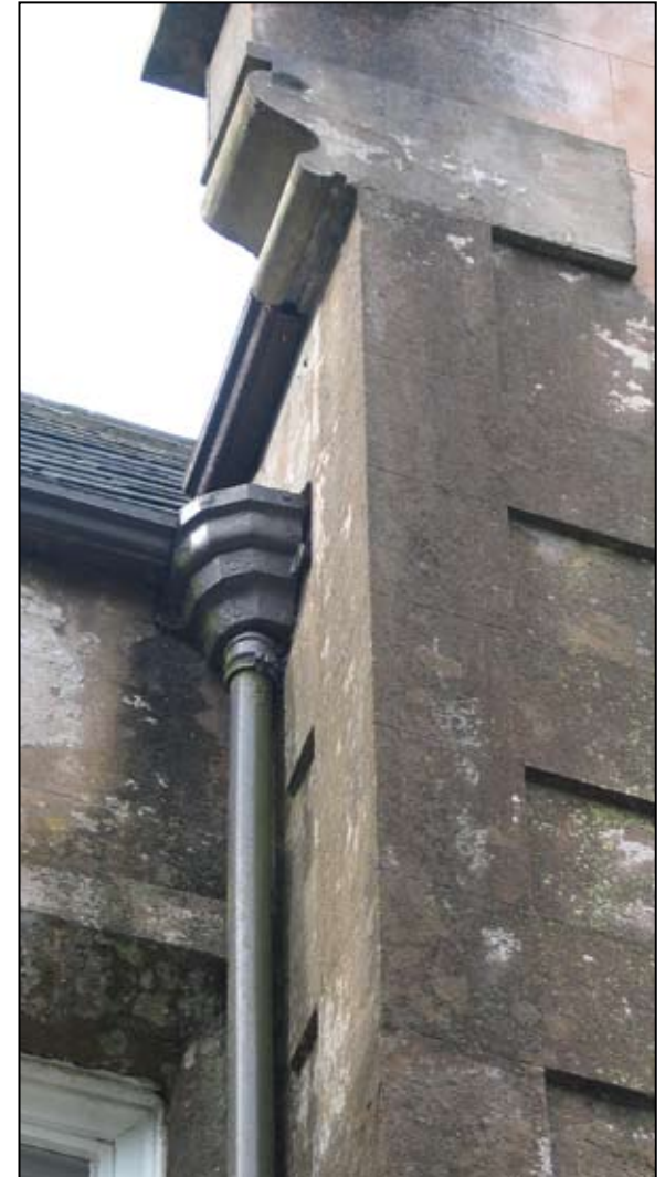
Cast iron rainwater goods
