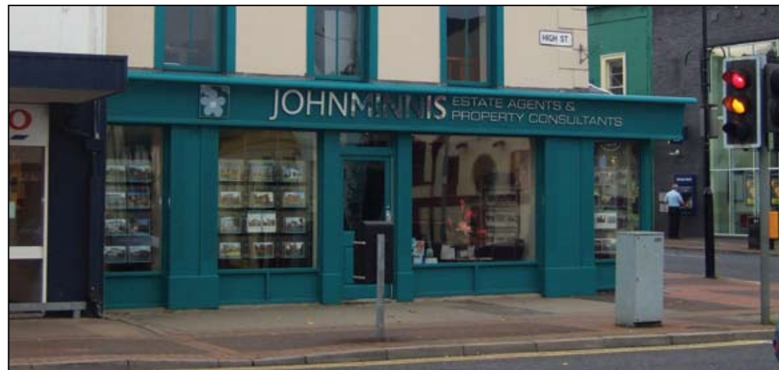
Shopfront, no. 44 High Street, Hollywood
