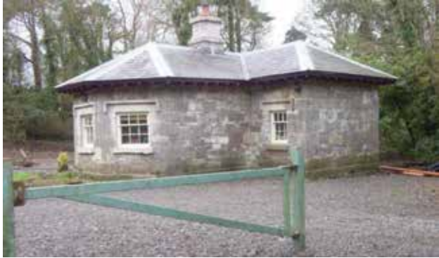
Ulster Canal Lock keepers cottage 601 at Tollymore Etra, Benburb, Co Tyrone prior to recent restoration
