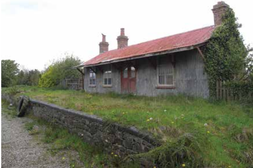
Corrugated metal railway station, Ballymagorry, near Artigarvan, Co. Tyrone
