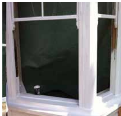
Repairs to outer linings and sill
