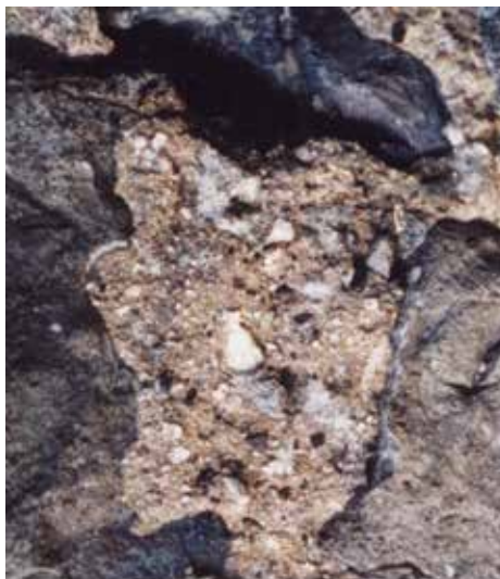
Lime Mortar, Rinndown Castle — note the coarse grain of the mortar.
