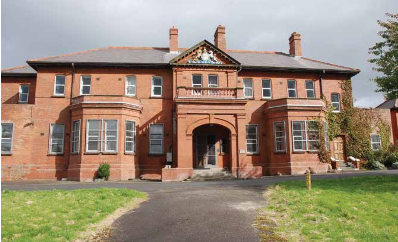
Former Officers' Mess, Ebrington Barracks, Londonderry
