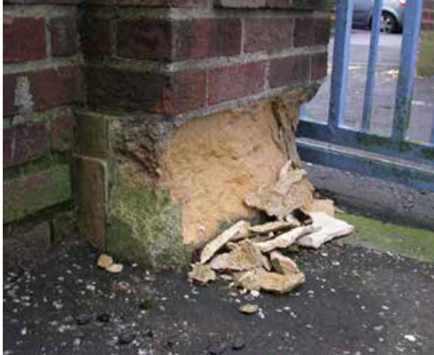
Collapse of a saturated sandstone block during the 'big thaw', which followed the 'big freeze' in December 2010 (Photo courtesy of D. McAlister)
