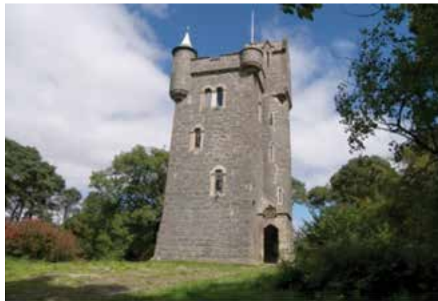
Helen's Tower, Clondeboye Estate, Co. Down
