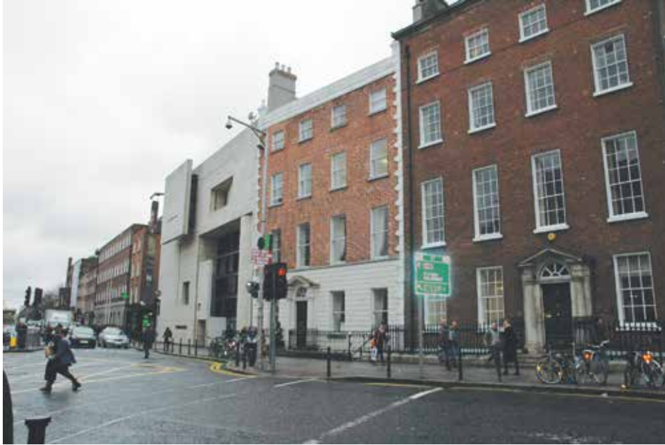
National Gallery of Ireland extension, Clare Street, Dublin, by Benson & Forsythe — considered successful and used as an example of good infill in the Department of the Environment Conservation Guidance document to Planning Authorities
