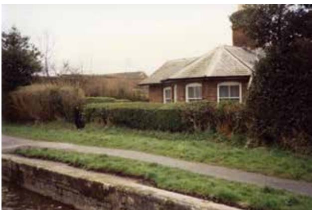
Lock keeper's cottage – Shropshire Canal – by Telford's offices
