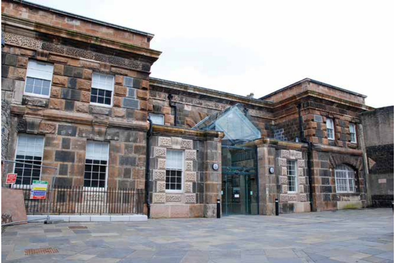
Rear of refurbished Gatehouse, Crumlin Road Gaol, Belfast
