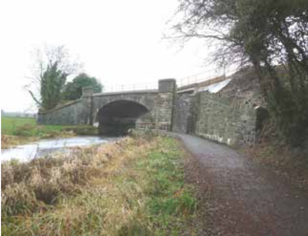
Railway bridge, Lagan Canal, near Moira, Co. Down
